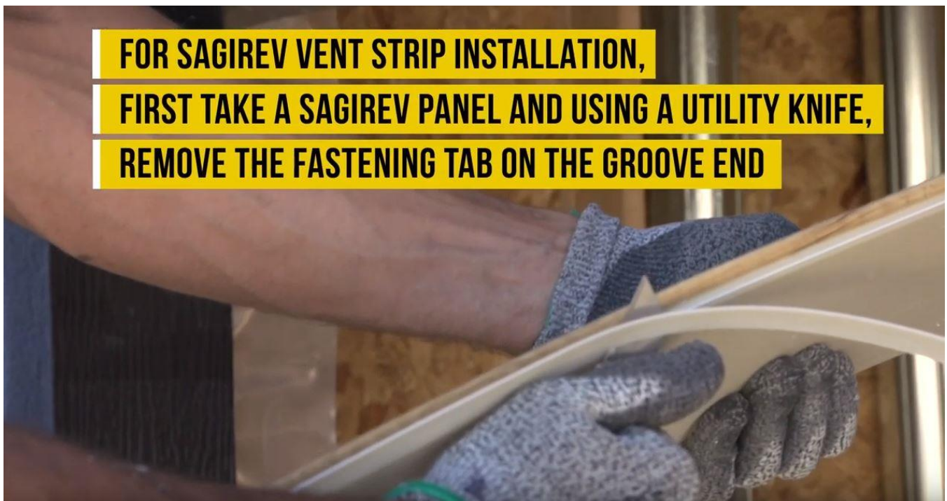
Figure 20, Remove fastening flange
