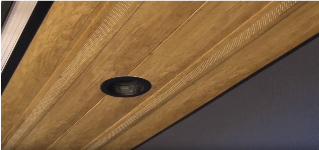
Figure 24, Soffit with light fixture
