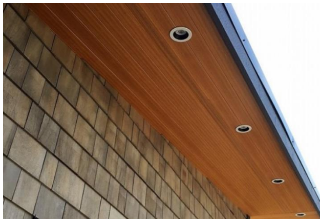
Figure 17, Soffit with SAGIREV Vent Strips, parallel application
