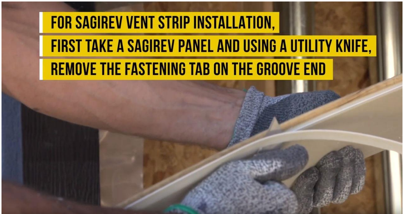
Figure 20, Remove fastening flange
