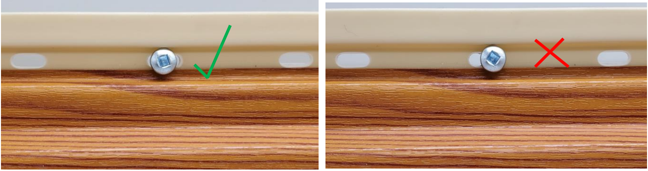
Figure 6.2, Fastening SAGIWALL Panels Top View
