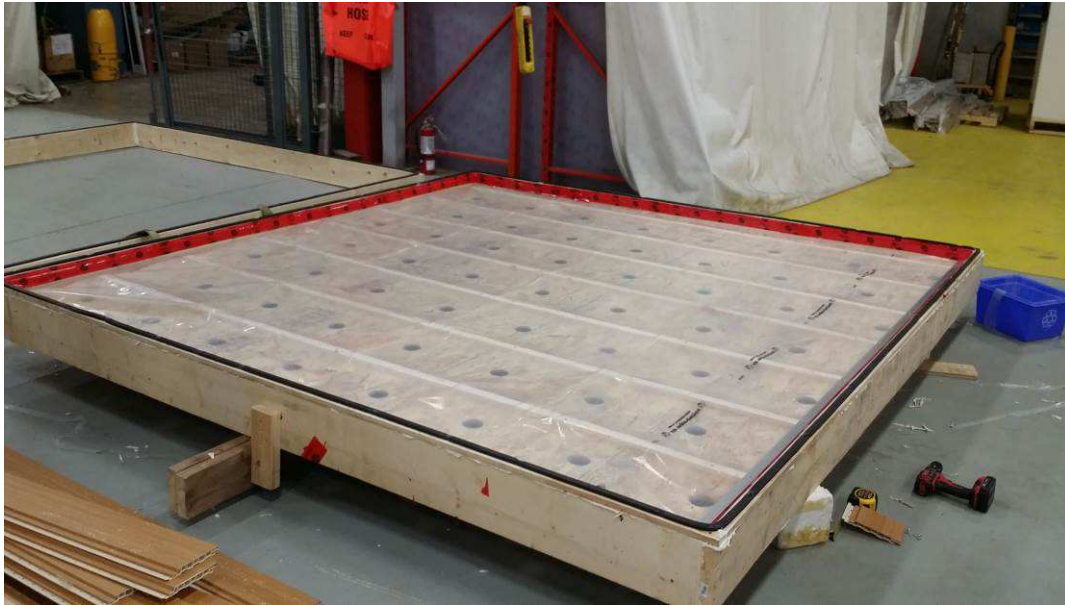
Figure A1 – Mock-Up Wall Construction
