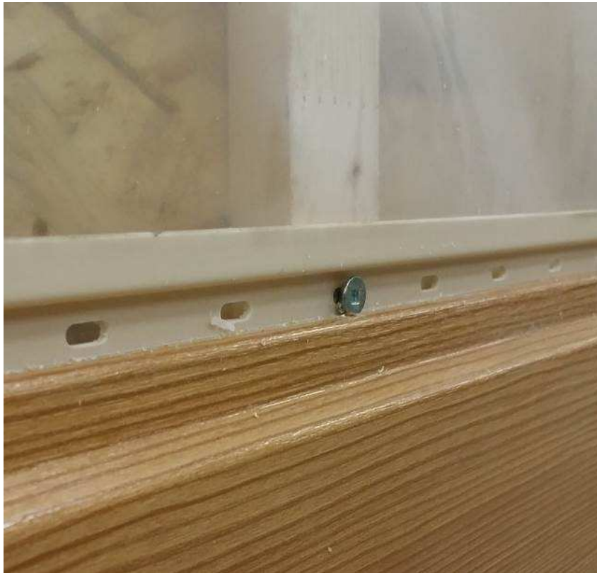
Figure A5 – Connection Point After Loading
